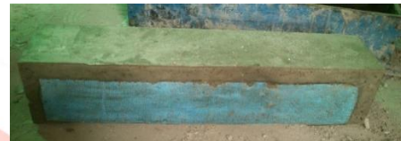
Fig 3: Casting of beam
