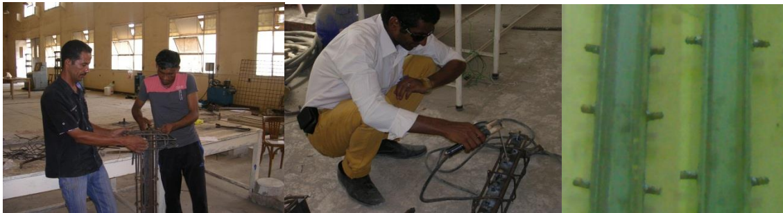
Fig. 3: Details of confining columns and shear connectors
