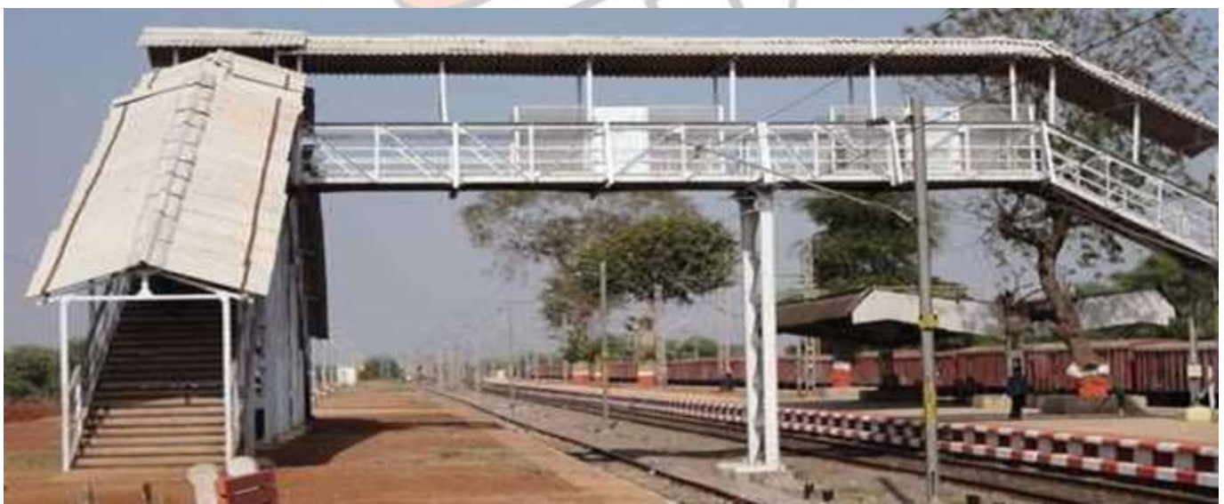
Figure 1: Foot Over Bridge.
