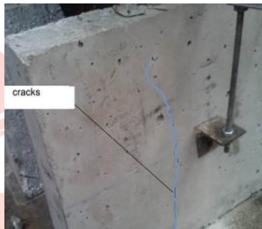
Figure (13): Failure of push-out specimen (P2)
