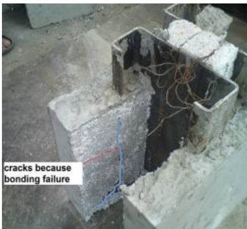
Figure (12): Failure of specimen (P1) without shear transfer enhancement.
