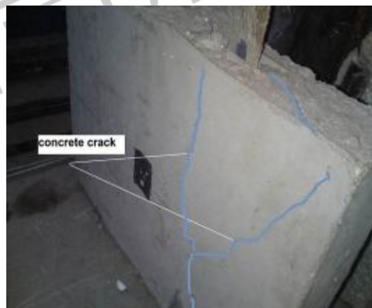
Figure (15): Typical cracking mode in push-out test specimen (P4).
