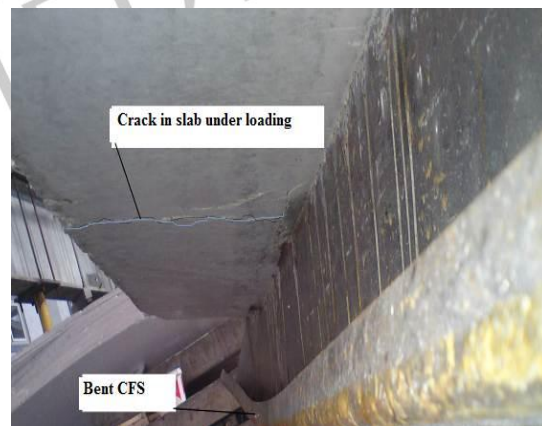
Figure (12): Typical large-scale test specimen (b2) failed due to concrete crushing.
