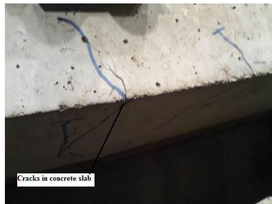
Figure(15): Typical large-scale test specimen (b7) failed due to concrete crushing.
