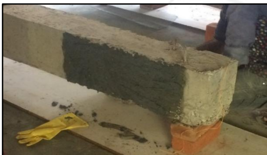
Figure 2 Shear Span Applied with MultiCrete Layer
