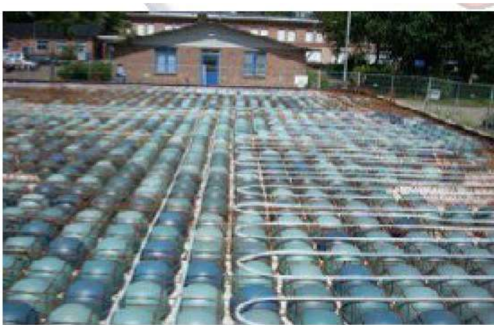
Figure 3: Installation of cooling or heating system
