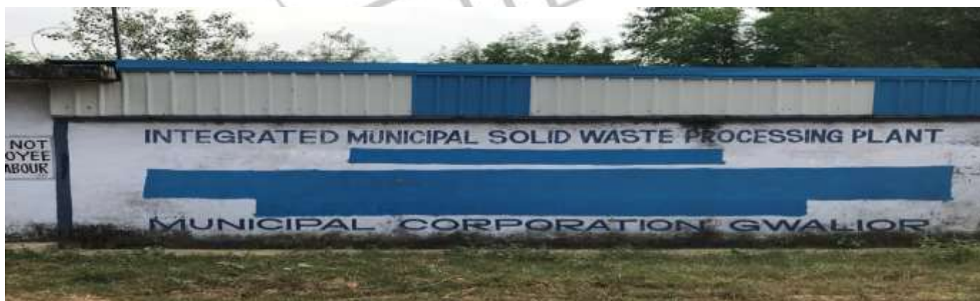
Municipal Waste Processing Plant, Gwalior.
