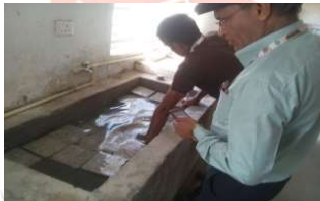
Figure 1. Curing of concrete
