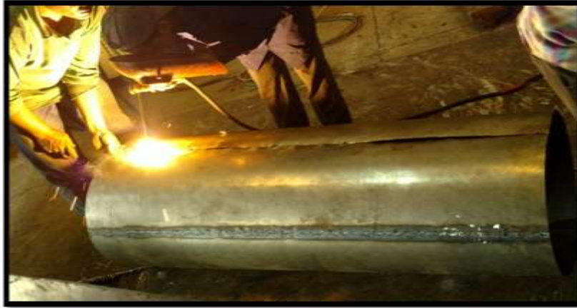
Figure 04: Fabrication of the pipe
