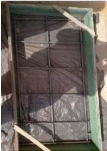
Fig. 6: Shape of Form work with reinforcement
