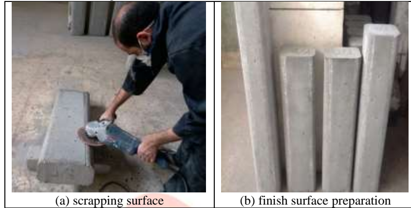
Figure 2. Preparing concrete surface
