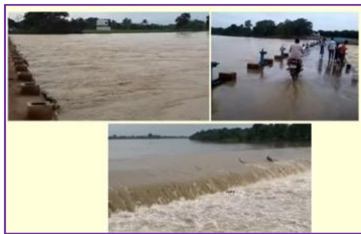
Fig. (5)- Flood in Shivnath (a)- water touching the bridge, (b)- water flowing over the bridge & (c)- water flowing over the bridge
