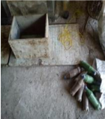
Fig.b.1- Wooden frame work
