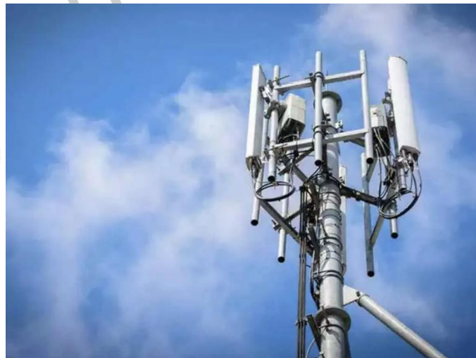
Figure 01: RRU & Telecommunication tower setup in real life
