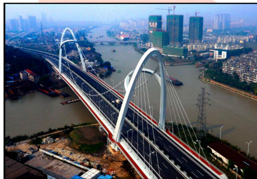
Fig. 3 – General view of Dongtiao River Bridge
