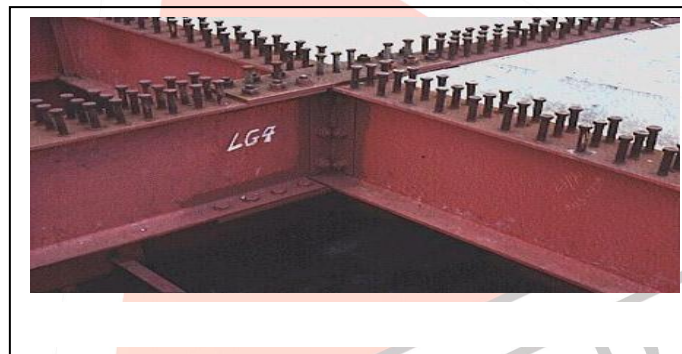
Fig. 2. Flexible type shear connectors
