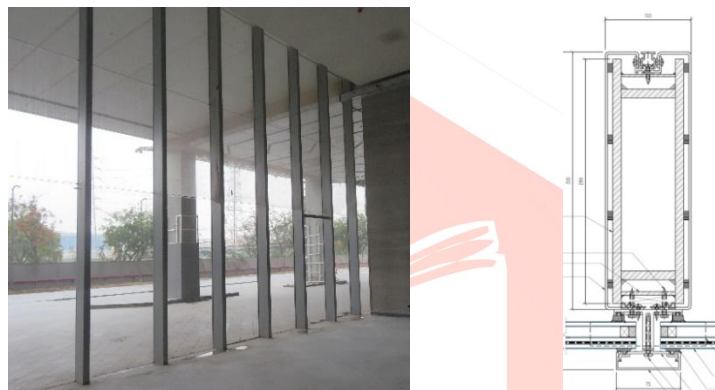
Figure 5: Triple height stick curtain wall system-Actual site installation view
