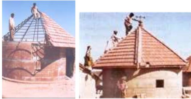
Figure 12: Construction of Stabilized Compressed earth blocks at Bhunga
