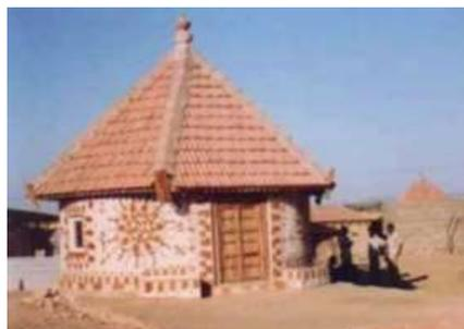
Figure 11: Stabilized Compressed earth blocks Bhunga
