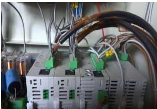
(Fig. 29) Controller of Plc. Circuit
