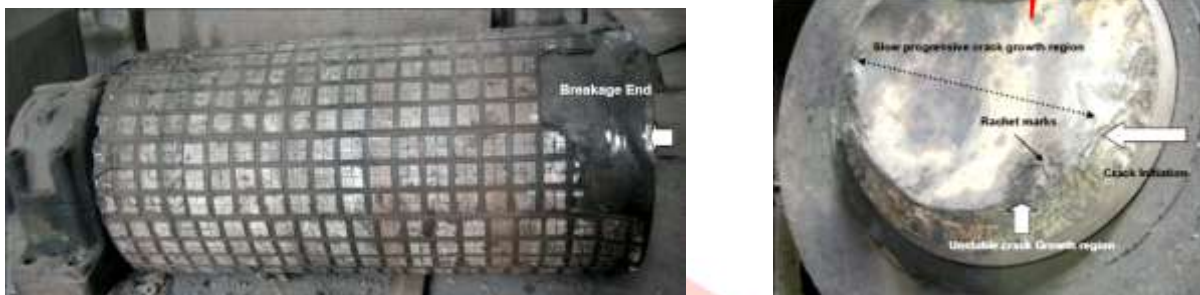
Fig. 1.1: Bend Pulley and its fracture Surface
