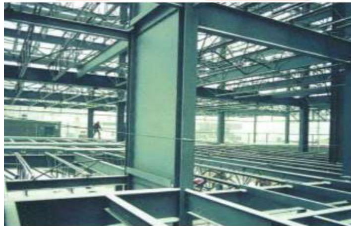
Fig.1 Unstiffened steel plate shear wall
