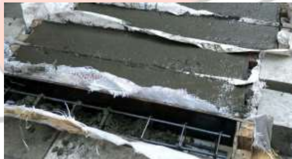
Fig (c): Beams After Casting
