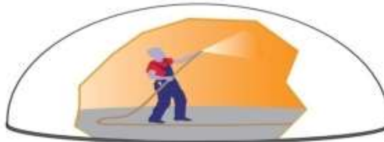
Figure .3- Application of polyurethane foam
