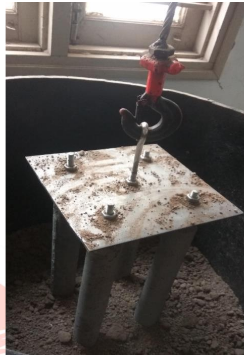
Fig 3.2.2 the setup of group pile
