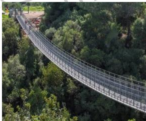
Fig.1. Simple Suspension Bridge.
