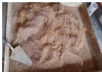
Fig 4.3 Mixing of soil cement and fibers
