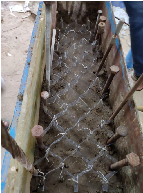
Fig. 5 Placement of geocell
